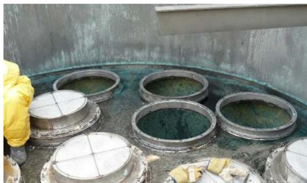
**Figure 3.** Hanging type mist eliminators being retrofitted with top meshpads.
