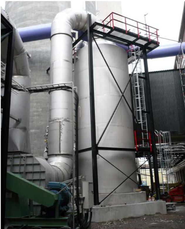
**Figure 1.** AN prilling tower candle filter system vessel.
