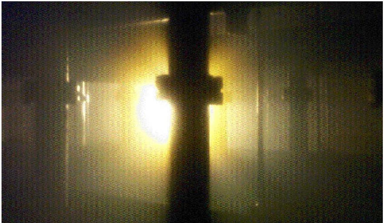
View through a sight glass below I.A.T. filters, showing normal inlet mist load
