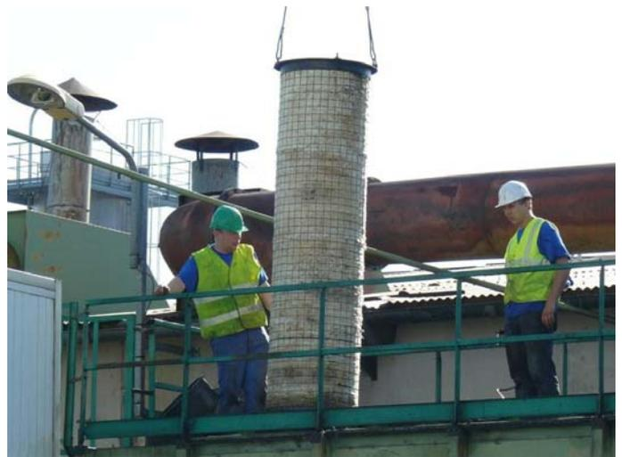
**HT2 Candle Filter being lifted for inspection**
