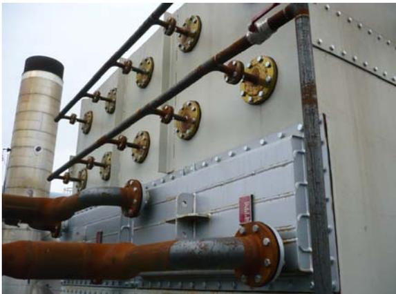
**Drawer-type Heat Exchanger Cooler below Pre-Filter Irrigation Spray Bar Connections**
